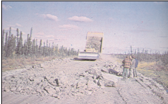
Access road under construction.
