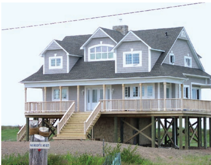
FIGURE 18: Construction of buildings on pylons as an example of adaptation that reduces vulnerability to storm surges, Grand-Barachois (near Shediac), Northumberland Strait, southeastern New Brunswick. Photo courtesy of Armand Robichaud.
