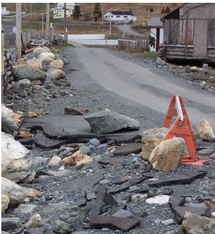
FIGURE 27: Storm-surge damage to road, April 2004, Ferryland, NL.
