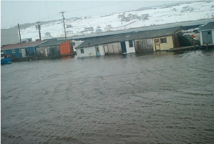
FIGURE 23: Flooding in St. Lawrence, NL., due to storm surge from Placentia Bay, February 2004, triggered by southwesterly wind (from Southern Gazette, Marystown, NL).
