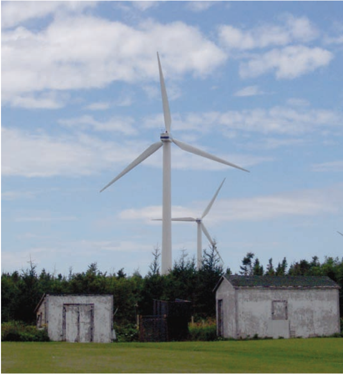
FIGURE 28: Experimental wind farm, North Cape, PE.
