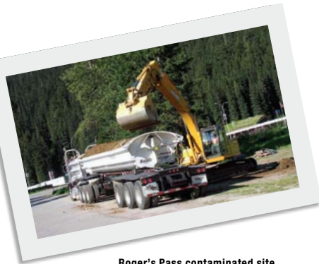
Roger's Pass contaminated site clean-up, Glacier National Park ©Parks Canada
