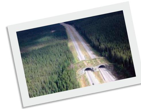
Wildlife crossing structure on the Trans-Canada Highway in Banff National Park ©Parks Canada
