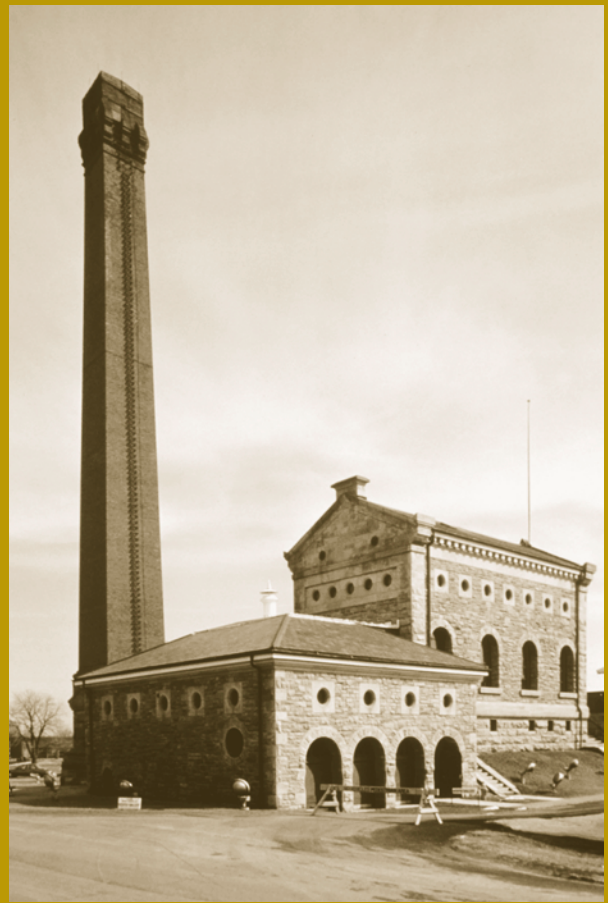
The Hamilton Waterworks, built in 1857-59, is the only intact mid-19 th century waterworks in North America. The character-defining compound-beam steam pumping engines were restored to working condition in 1998.
