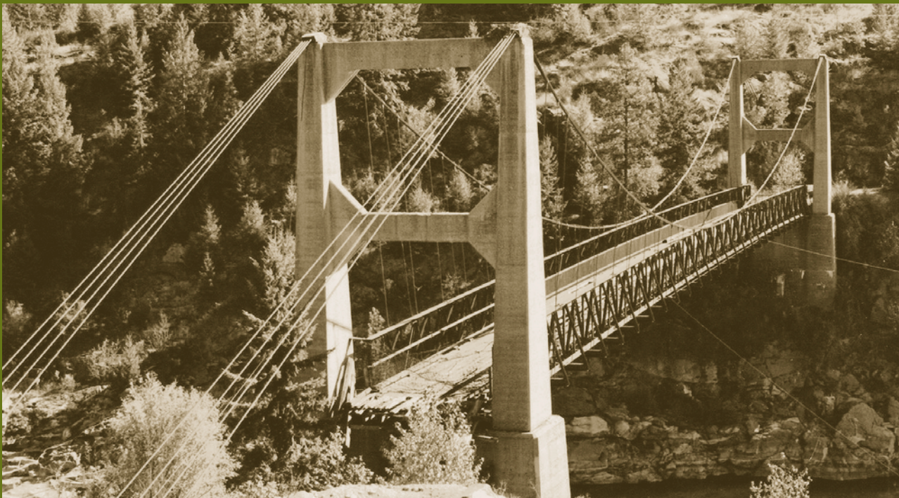
The Brilliant Suspension Bridge was built over the Kootenay River near Castlegar, British Columbia in 1913. Ensuring public safety is one of the primary concerns of professional engineers.
