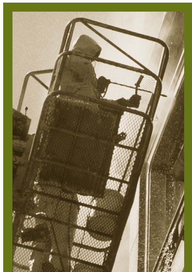
Trained and skilled workers are a vital part of a well-thought out and well-executed conservation project.
