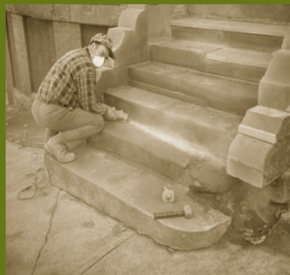
In Rehabilitation , deteriorated features should be repaired, whenever possible, and replaced when the severity of the damage makes it necessary. Here, the character-defining stone steps of the entrance to a house in Saint John, New Brunswick were cracked. Appropriate work on the entrance included repairs to the stone steps and walls, and the installation of a metal handrail to meet building code requirements.
