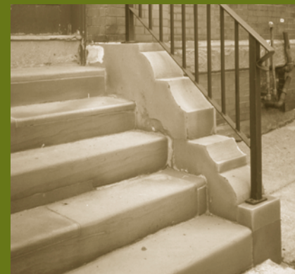
In Rehabilitation , deteriorated features should be repaired, whenever possible, and replaced when the severity of the damage makes it necessary. Here, the character-defining stone steps of the entrance to a house in Saint John, New Brunswick were cracked. Appropriate work on the entrance included repairs to the stone steps and walls, and the installation of a metal handrail to meet building code requirements.
