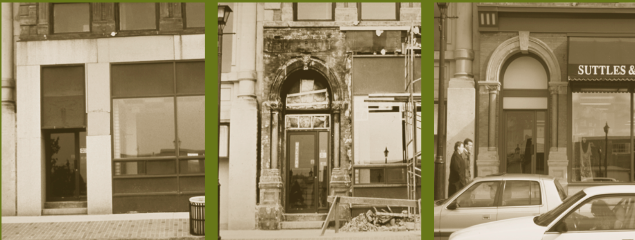
Restoration of a storefront may involve removing inappropriate cladding dating from a later period. Recreating a missing feature, such as the awnings on this storefront in New Brunswick, should be based on physical or documentary evidence.
