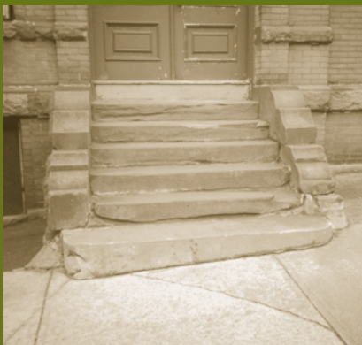
In Rehabilitation , deteriorated features should be repaired, whenever possible, and replaced when the severity of the damage makes it necessary. Here, the character-defining stone steps of the entrance to a house in Saint John, New Brunswick were cracked. Appropriate work on the entrance included repairs to the stone steps and walls, and the installation of a metal handrail to meet building code requirements.
