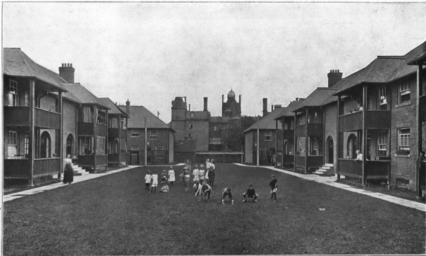
Spruce Court. Partial view of The Toronto Housing Company's Property on Spruce Street.
