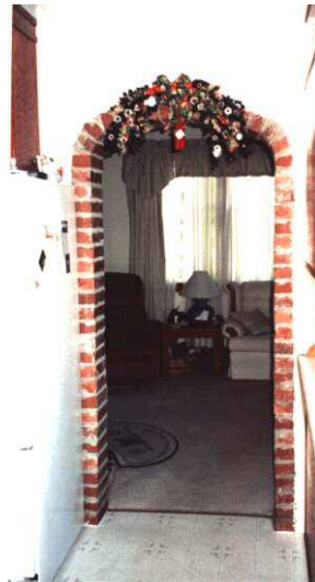
Figure 24 A recent transformation of a brick chimney.
