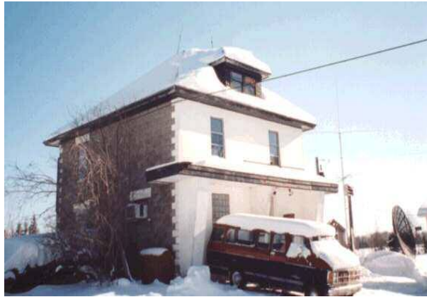
Figure 12 Ambrose WHEELER, former mayor of Moncton, owned this property before it was purchased by Moncton Broadcasting Company. (Demolished)
