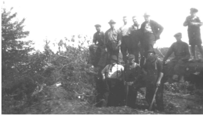
Figure 45 A work crew clearing shrub at McNutt Brook. Far left in front row is T. E. FITZSIMMONS.
