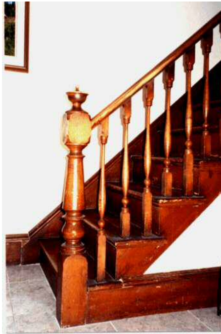
Figure 14 The original staircase as seen in spring 2002.
