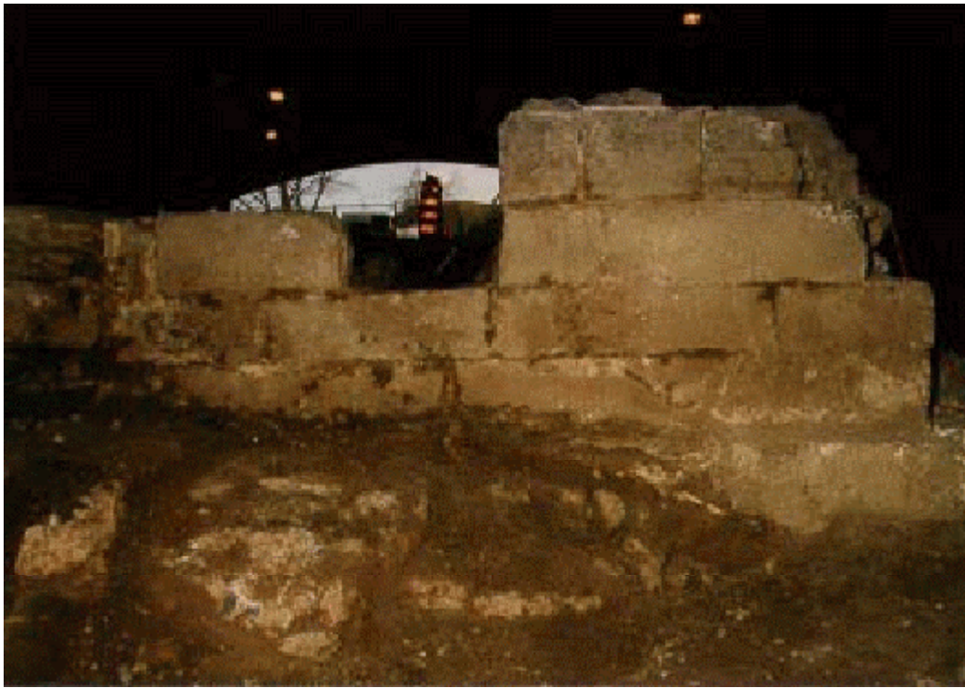
Figure 12. Remains of the north face of the Sappers' Bridge on a bedrock outcropping as found in February, 1998. The four courses of dressed ashlar to the right remain and are now displayed in situ . (Parks Canada photo by J.-P. Jérôme; J-2/10)
