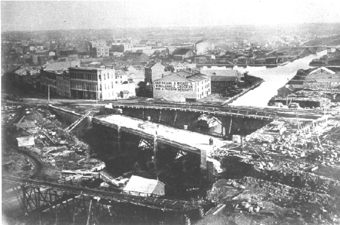
Figure 4. "Dufferin Bridge during the course of construction, ca. 1874". The Sappers' Bridge is also being widened and the new cut through its masonry for the road is not yet completed. (Public Archives of Canada; C493).
