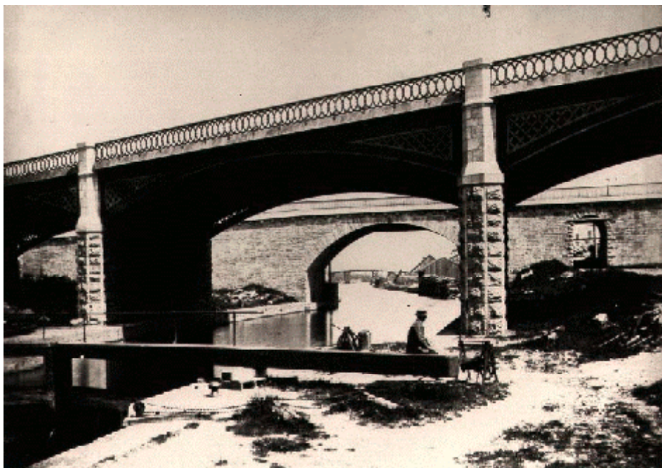
Figure 5. "Under Dufferin Bridge, Looking South" 1882. The new opening through Sappers' Bridge masonry is visible on the left. (Public Archives of Canada, 9306).
