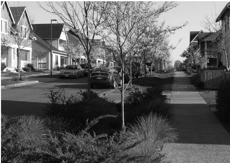
Bioswales line a street in West Seattle, Washington to enhance infiltration and reduce runoff.
