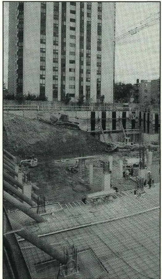
A downtown Toronto construction site
