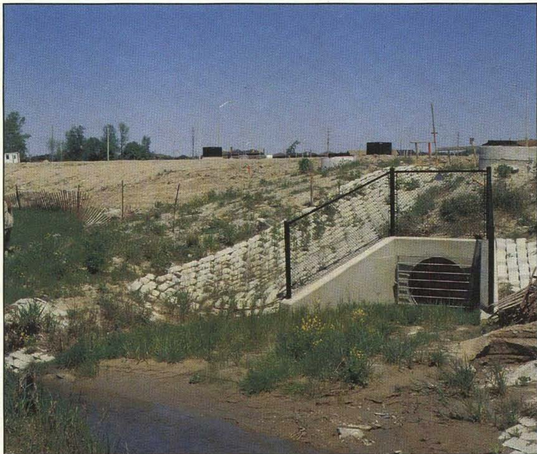
A typical storm-sewer outfall
