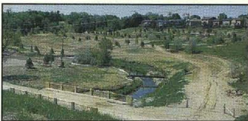
Golf course under construction
