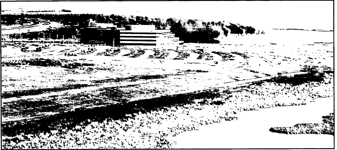
General Motors headquarters building near the Oshawa Second Marsh
