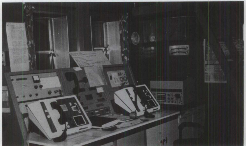
2.10 The Ocean Ranger's radio room contained the primary communications equipment, installed in this console. The two inclinometers in the corner of the room were similar to those installed in the ballast control room and several other locations.
