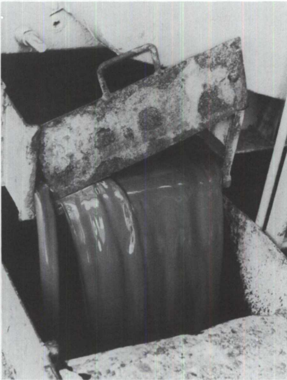
FIGURE 5 Drill fluid being pumped from the J-34 well.
