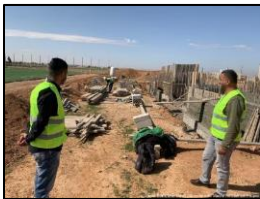
Image number 6: two workers on a construction site.
