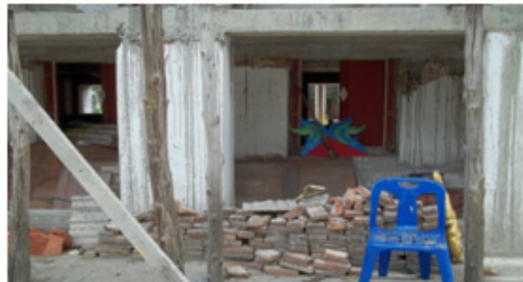
Figure 5. Merger of the old and new temple walls
