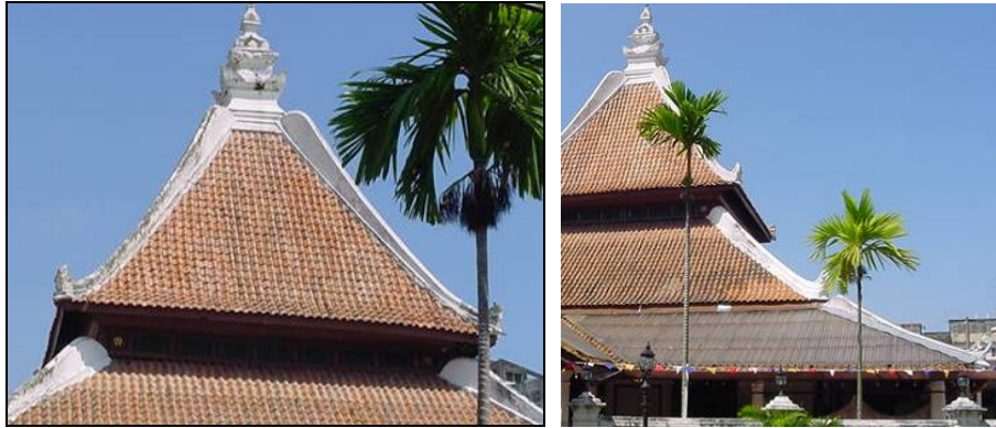
Figure 4. Pyramid roof shade (left) and attached roof system (right)
