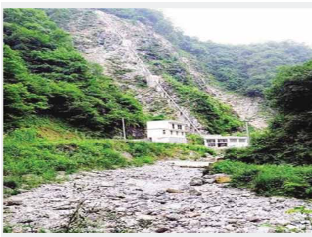
Figure 2. Dried bed of a stream just downstream of the diversion weir of a SHP
