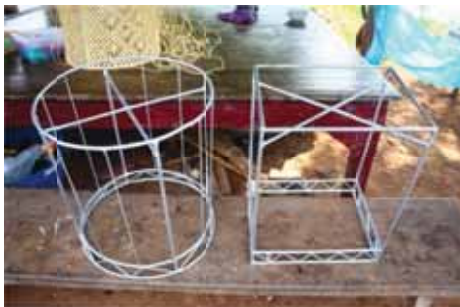
Figure 2. Cut and solder metal pieces into frames for making weaves as designed
