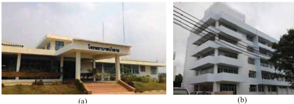
Figure 7. Photographs of (a) the OPD building and (b) the wards building
