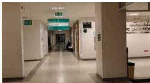
Figure 14. The current condition of the corridor intersection in front of the entrance to the blood test lab
