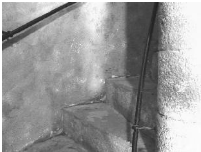
Fig. 9: Some of the 235 steps to the top.
