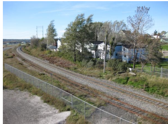
Figure 6: Pier houses next to plant.
