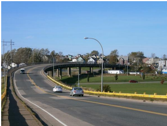
Figure 2: Bridge to Whitney Pier.
