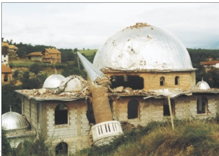
A demolished mosque and minaret in Prizren, Kosovo
