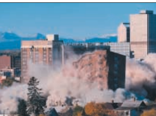
Ultimate restructuring: Calgary's Bow Valley Health Centre was demolished in October 1998
