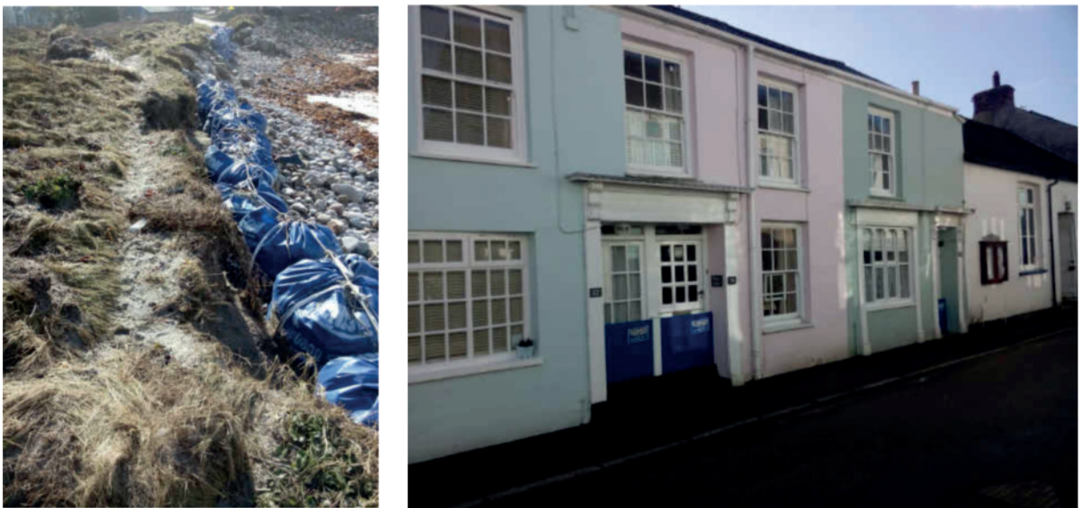
Figure 10: Stabilisation of dyke on St Agnes (left); flood boards in front of holiday flats in Flushing (right).
