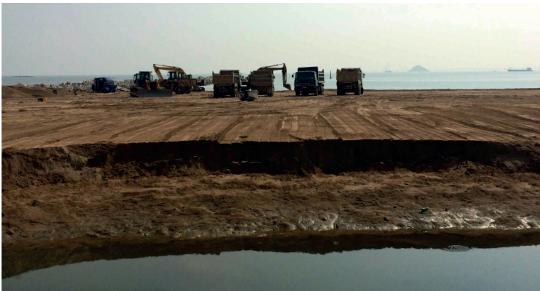
Figure 5: Xianglu Harbour beach, under renovation in December 2015. (Source: © Hong Gang, 2015.)
