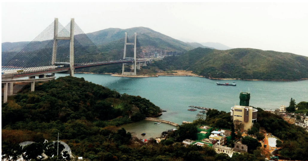
Figure 3: A series of bridges connect the peripheral islands of Lantau Island, Ma Wan, and Tsing Yi to the urban core of Kowloon and Hong Kong (Photo taken at Ma Wan). (Source: © Abraham Leung)
