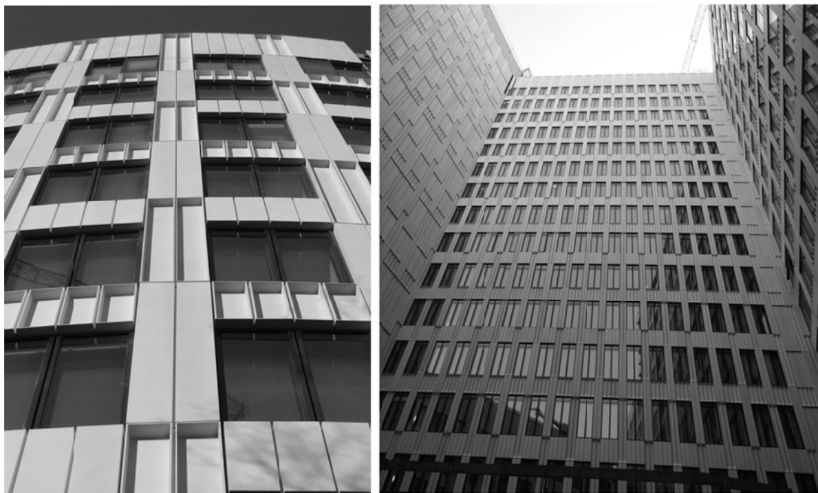
Figure 5. Mounted façade elements on the multistory building “Leo”
