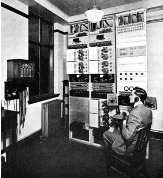
Figure 3. Interior of CNR radio control room (McDowell, 1932, p. 8).
