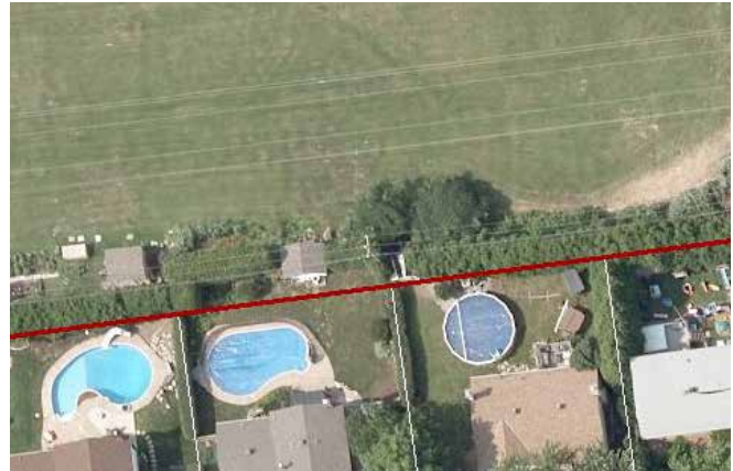
Examples of properties that encroach (above the red line) on the land identified under the Order / Photo: © Environment and Climate Change
