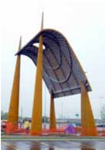
John McEwen's Heaven and Earth under construction at the Cineplex Odeon movie theatre at Islington and Queensway in Toronto. Photo courtesy John McEwen.
