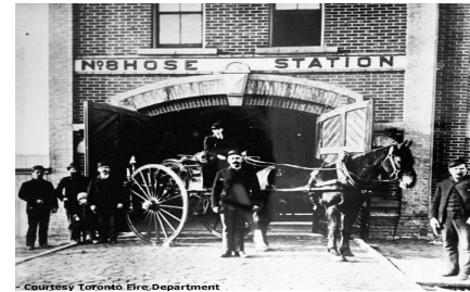
No. 8 Hose Station
