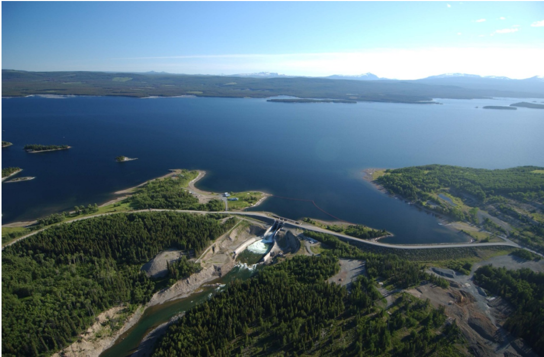
Figure 10: The Skins Lake Spillway 279
