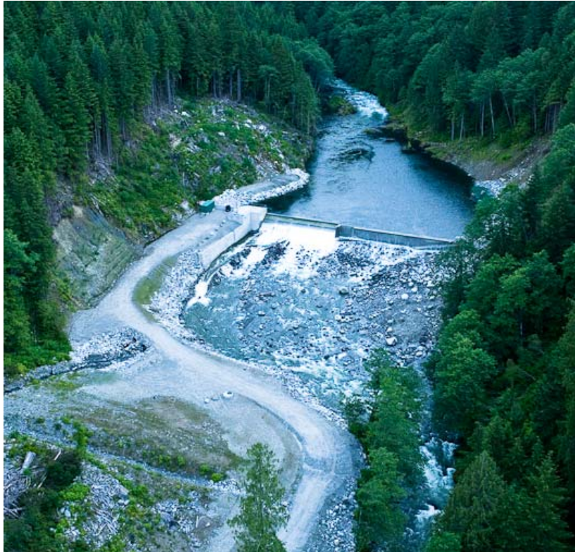
Figure 24. Intake and headpond of the Douglas Creek generating station (a typical installation). The intake weir creates a headpond and raises the water so a portion of stream flow can enter the penstock. The size of the headpond is determined by the topography at the intake location. This installation is upstream of an alluvial fan on which Harrison -downstream migrating-Late timing sockeye salmon spawn (image from http://cloudworksenergy.com/projects/photo-tour/ ).
