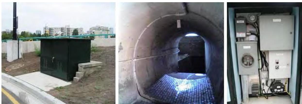
Heather CSO kiosk, sampling tube installation in Balaclava CSO and kiosk electronics
