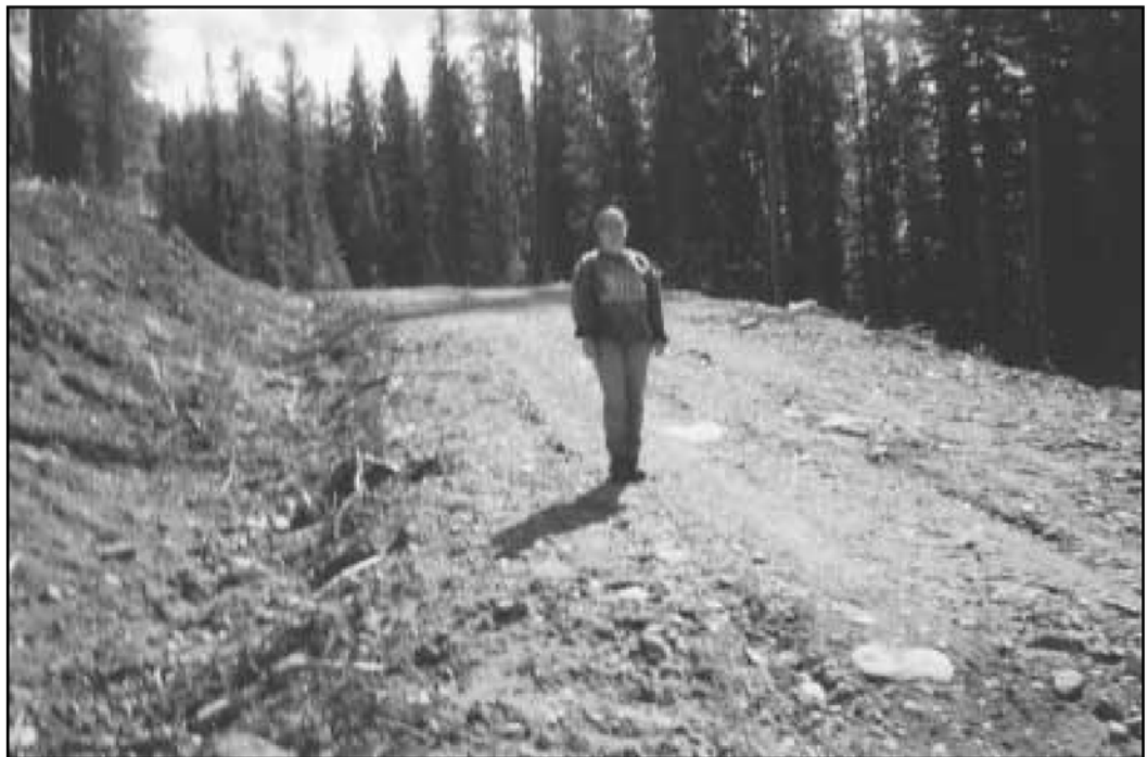
Figure A3.4. Example of sediment production class 4 (sediment production = 70 \text{ m}^3/\text{km}/\text{yr} ).
