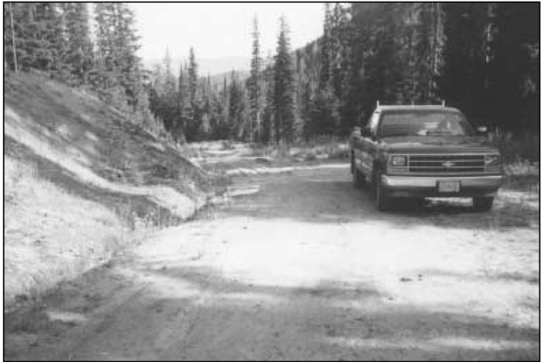
Figure A3.4. Example of sediment production class 4 (sediment production = 70 \text{ m}^3/\text{km}/\text{yr} ).
