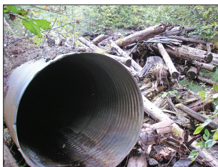
FIGURE 7b Deactivated road crossing debris in stream channel at "Craze Creek" upper-basin site, logged 1977.
