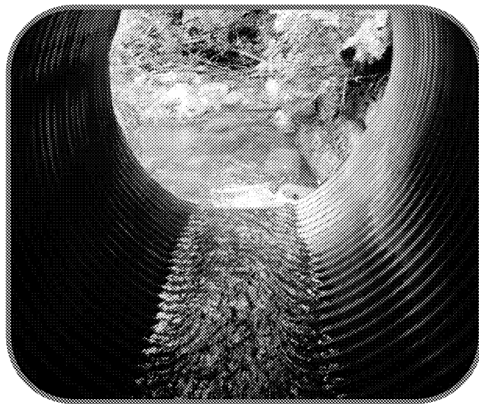
FIGURE 11. An example of a CBS culvert on an important habitat fish stream. The outlet drop and the length of the culvert, with no velocity refuge, is a partial impediment to fish passage.
