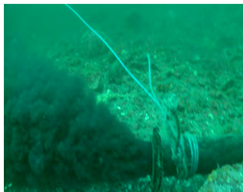
Figure 3. Farm salmon processing plant 12" out-fall pipe at 90', showing blood water (containing west Vancouver Island sea lice eggs) which appears black at this depth photo by Twyla Roscovich.
