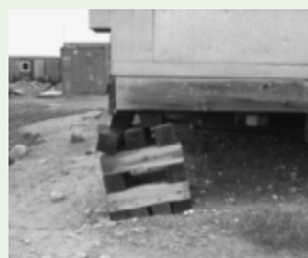
Thawing of permafrost causes uneven shifting of building's foundation
