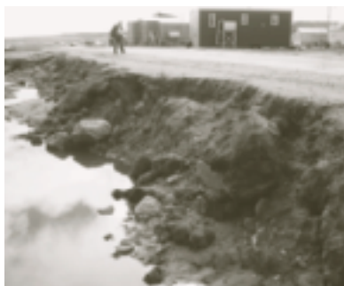
Erosion of permafrost that undercut a road Photo: Natural Resources Canada
