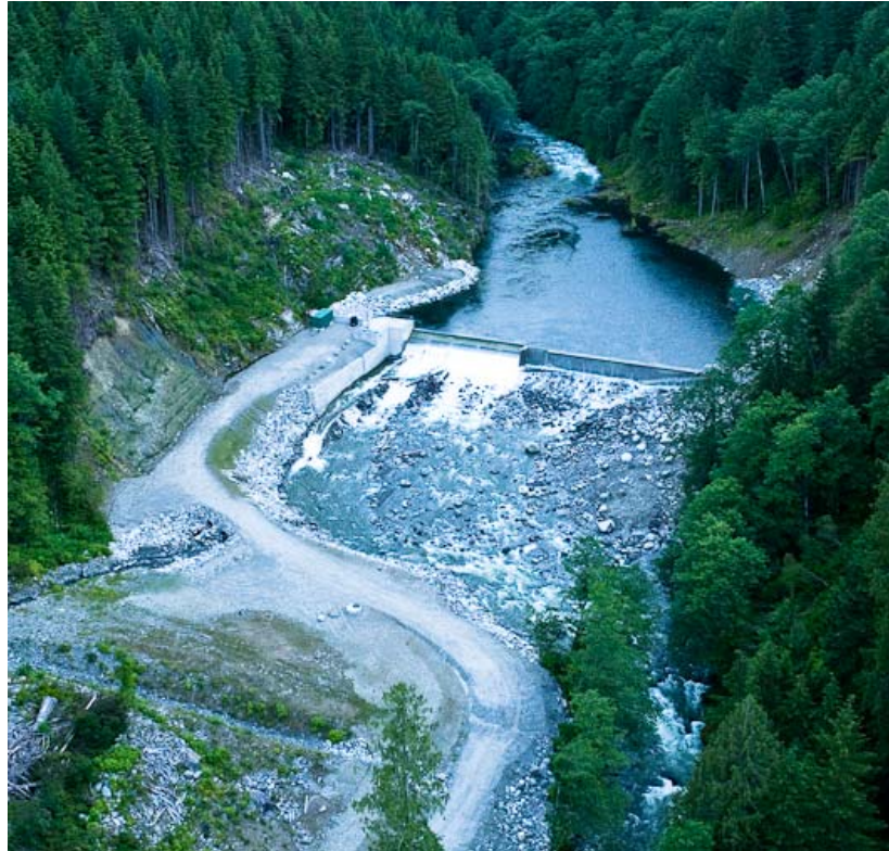
Figure 24. Intake and headpond of the Douglas Creek generating station (a typical installation). The intake weir creates a headpond and raises the water so a portion of stream flow can enter the penstock. The size of the headpond is determined by the topography at the intake location. This installation is upstream of an alluvial fan on which Harrison -downstream migrating-Late timing sockeye salmon spawn (image from http://cloudworksenegy.com/projects/photo-tour/ ).
