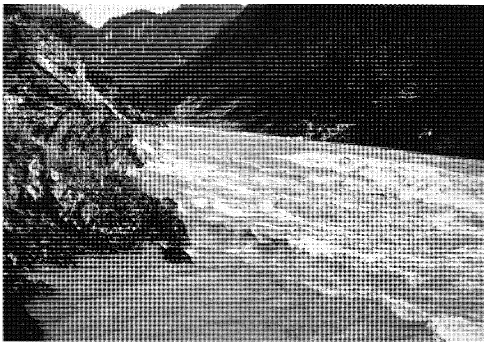
FIGURE 3B—A picture of the Fraser River taken after the removal of the rock pinnacle shown above, illustrating the successful removal of the obstruction.
