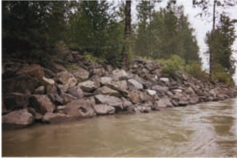
Figure 3-18. Examples of bank armouring along the Fraser River in the gravel reach.
