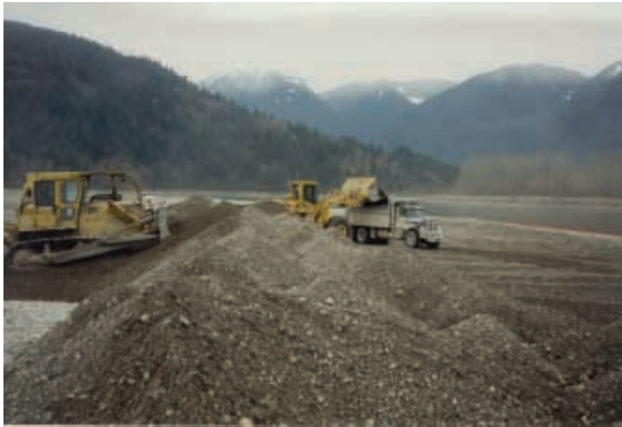
Figure 3-20. Transport of gravel excavated from Harrison Bar to the mainland across Minto Channel, February 2000.
